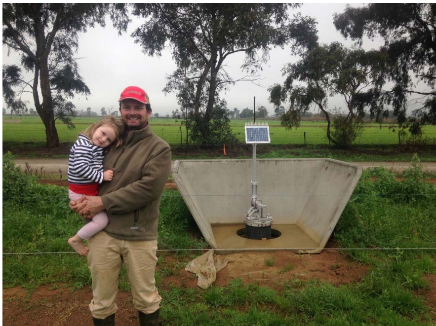
Proponent Nick Ryan and Daughter with their completed riser with blade valve, and I-Bee automation, Lancaster Vic.
